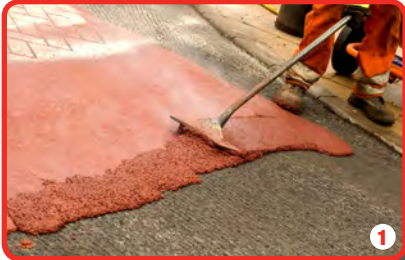
Hot Imprint material is spread evenly over the surface
