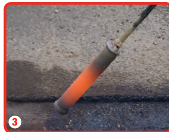
3 Thermal lance is used to remove moisture and debris
