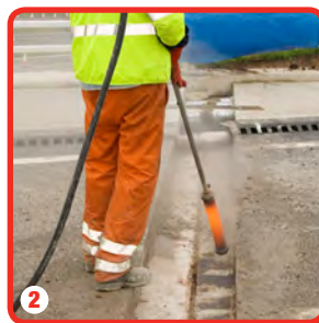
2 Preparing the recess
