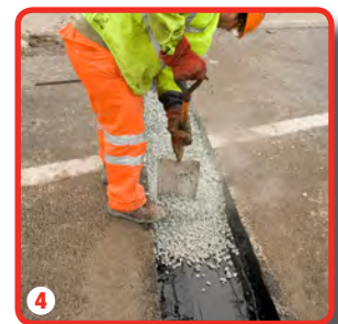
4 Applying first layer
