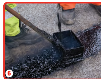
6 Filled crack is screeded over with Fibrescreed RC100MTR bitumen to create a watertight seal
