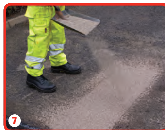
7 Aggregate is broadcast over the surface to provide an appropriate skid resistance level
