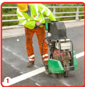
1 Cutting the recess
