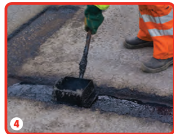
4 Base of recess is sealed with Fibrescreed RC100MTR bitumen
