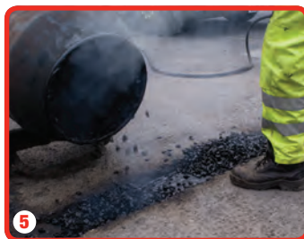
5 Fibrescreed RC100MTR stone/bitumen topping mix is added (if required depending on planed depth)
