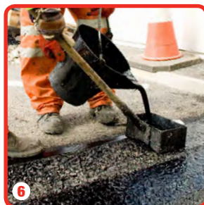
6 Applying finishing layer
